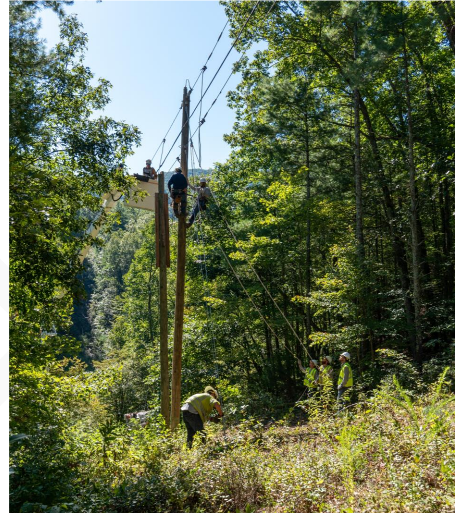
Crews complete make ready work in Botetourt County, Va
